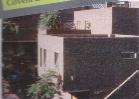
GLC built new homes in central London at Odhams Walk, Covent Garden
