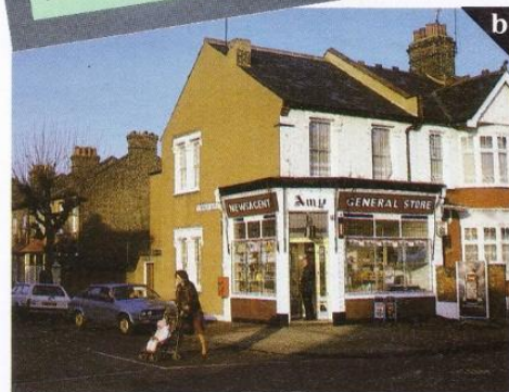
Protecting local shopping: a derelict shop in Wandsworth a
